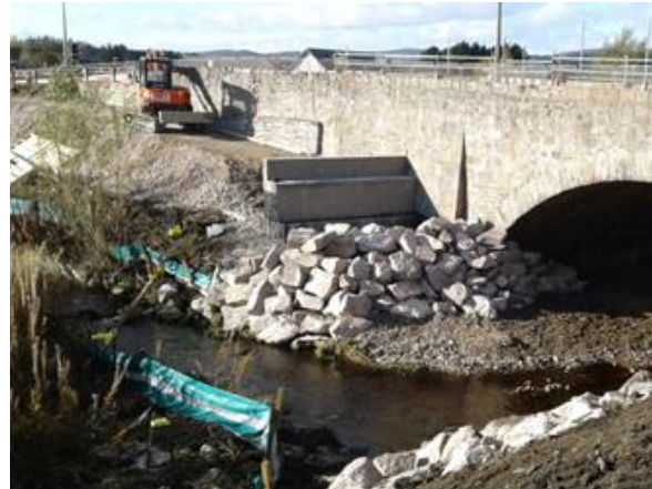
Figures 54 & 55 – retained riparian habitat and sediment management in place during construction,
