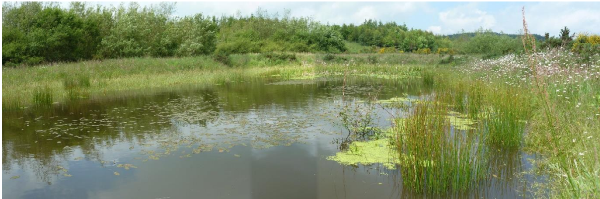
Figure 42 – an example of an appropriately formed and ecologically-rich SuDS design constructed within the A1 trunk road corridor at Houndwood. East Lothian.
