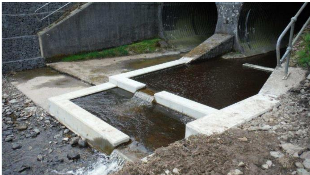
Figure 45 – retrofitting facilities like the artificial pools and weirs to ‘hard engineered’ culverts can introduce greatly improved habitat and species connectivity where barriers previously existed.
