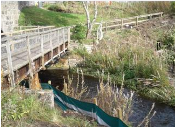
Figures 54 & 55 – retained riparian habitat and sediment management in place during construction,
