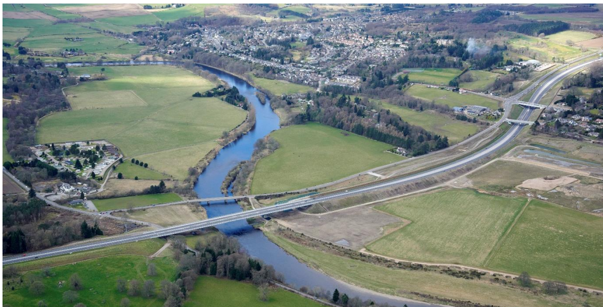
AWPR/B-T trunk road crossing at the River Dee
