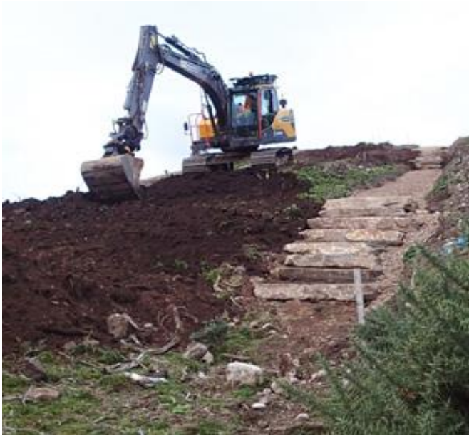
Installing stone steps at the John O'Groats Walking trail
