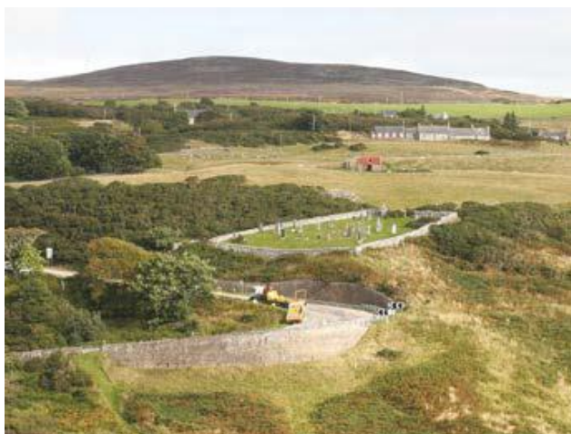
Existing road at Berriedale Braes
