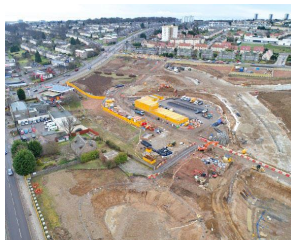
Progress on the Sustainable Urban Drainage System
