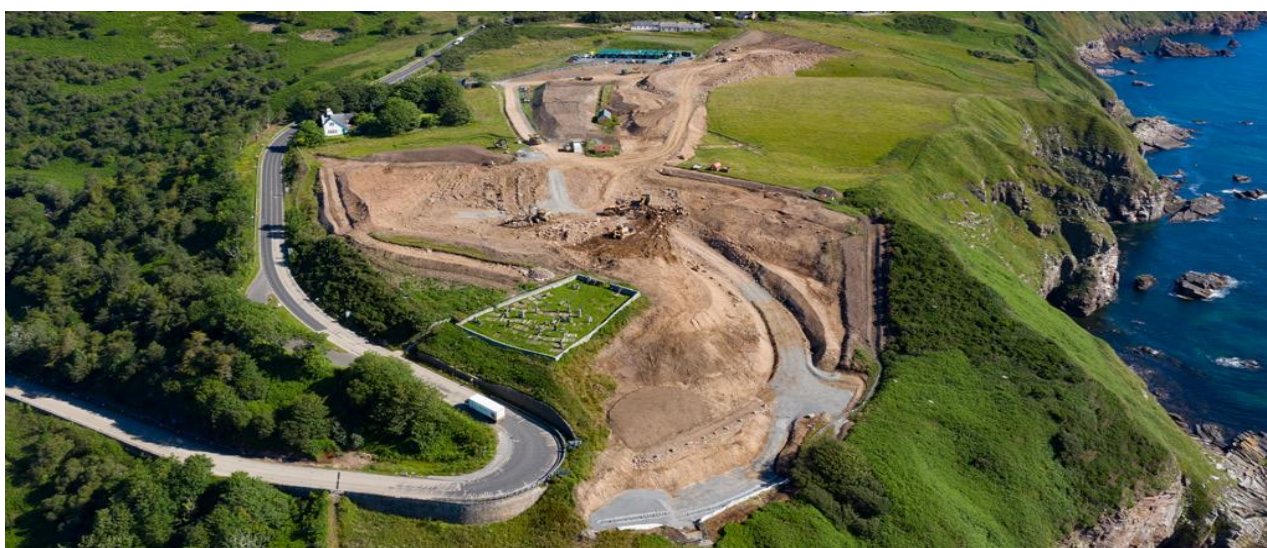
Aerial view of Berriedale Braes during construction
