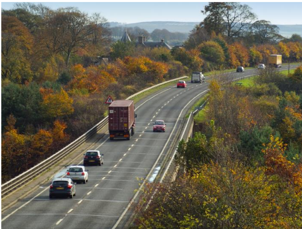
A96 at Inverurie at the River Don crossing looking towards Aberdeen
