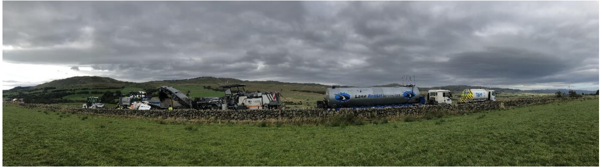
The in-situ recycling centre in operation
