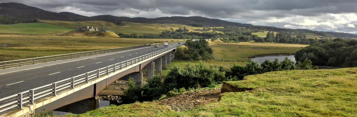
Lot 1 – Existing Spey Bridge with Rutherven Barracks
