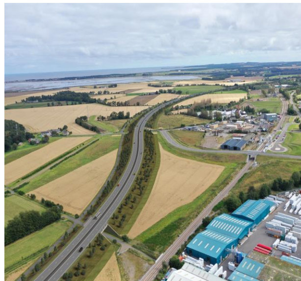
Artist's impression of proposed A96 dual carriageway at Forres looking North East.
