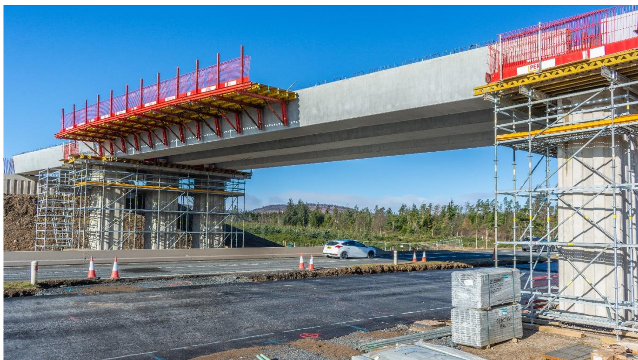
Concrete bridge beams in place on the Gelly Overbridge
