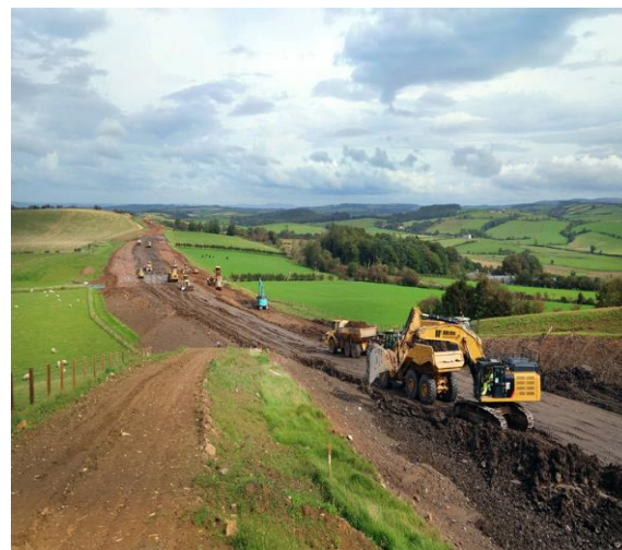
Work now underway on the Maybole Bypass
