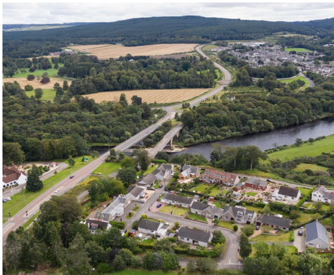
Existing A96 route approaching the River Spey looking East.
