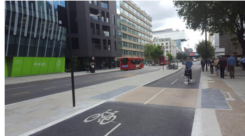
Example of an Active Freeway
