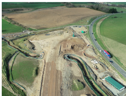
Smithston Roundabout at the northern tie-in
