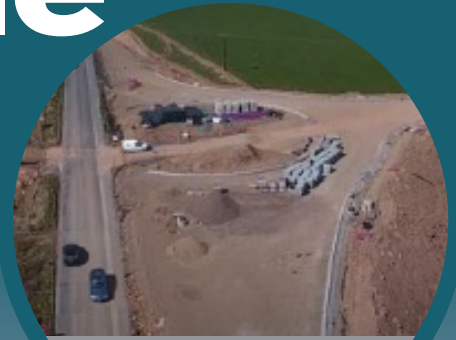
Roundabout at Culzean Road
