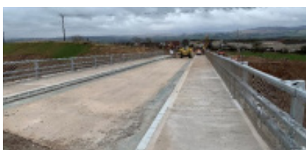
Footpath and parapet construction at Gardenrose Path
