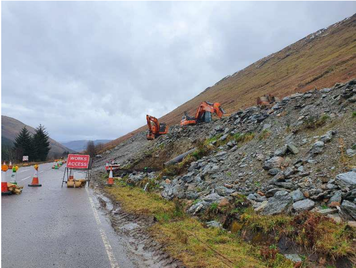
Image showing ongoing works at Glen Kinglas Bunds
