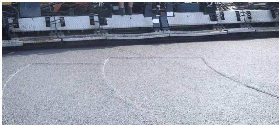
Figure NG 2.5 Roller compaction behind paver
