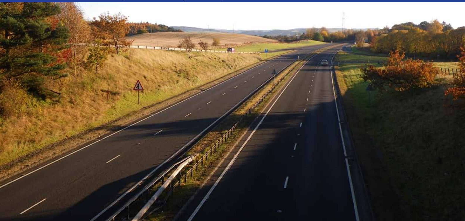
The A9 looking south from the bridge at Luncarty.
