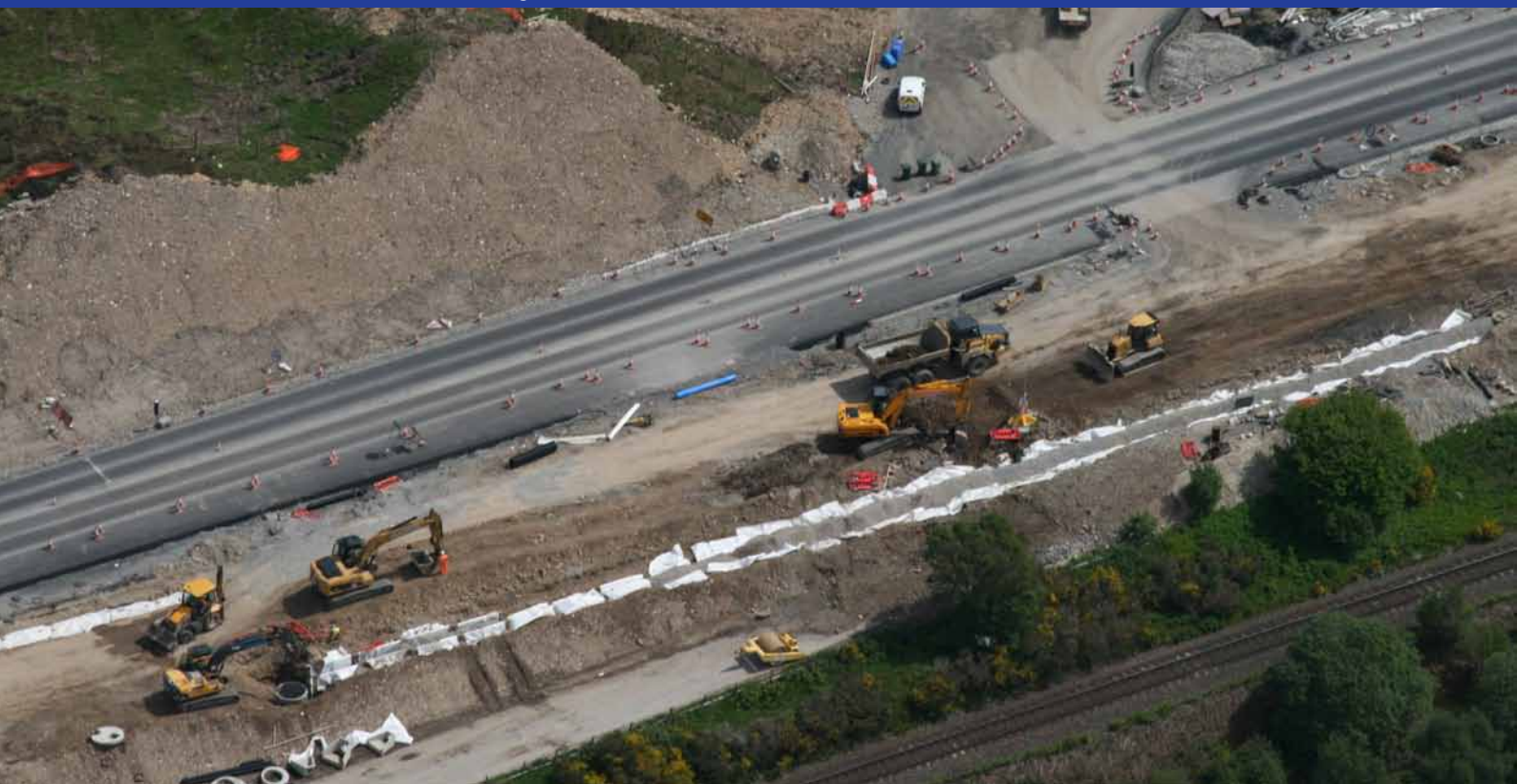
Construction of the dualling at Crubenmore.
