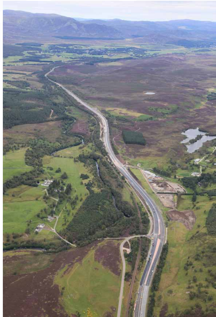
The A9 at Crubenmore looking north.
