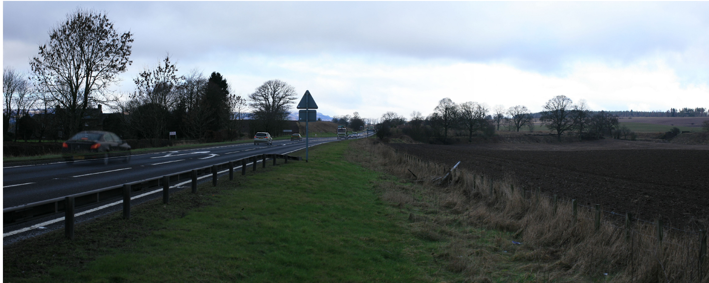
VIEWPOINT LOCATION 2 - Existing photograph looking north along A9 towards Newmill
