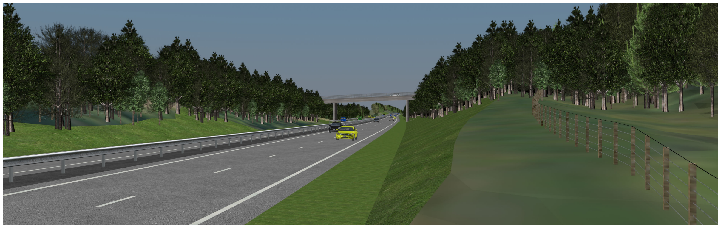
VIEWPOINT LOCATION 1 - VRM Still - Representative view looking south along proposed A9 alignment towards Pitlandie Overbridge
