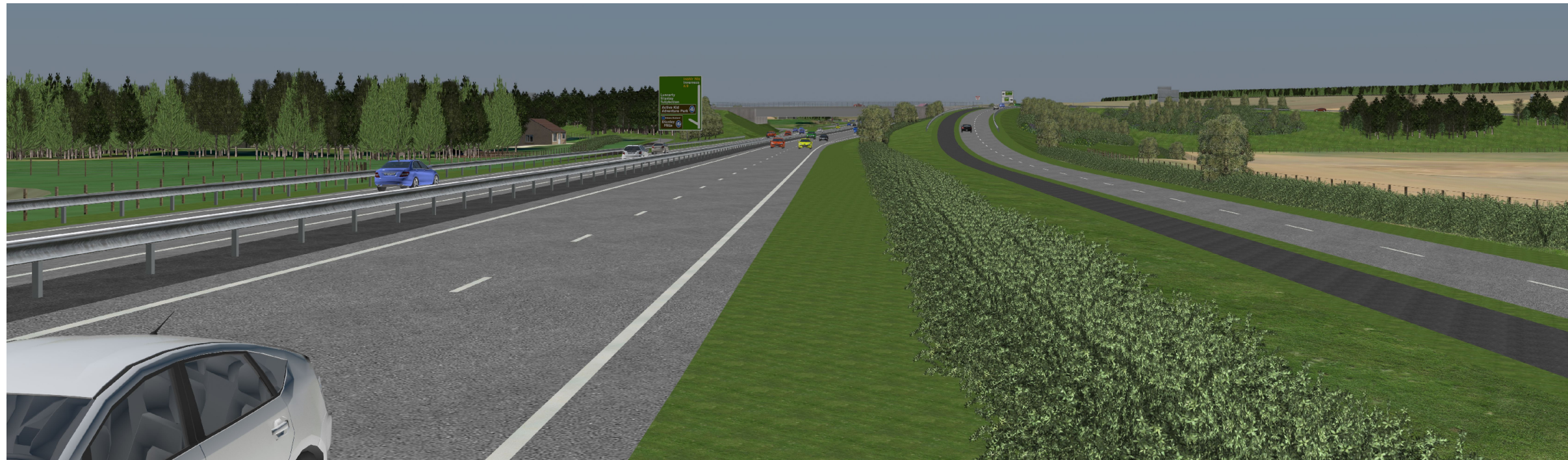
VIEWPOINT LOCATION 2 - VRM Still - Representative view looking north along proposed A9 alignment towards Tullybelton / Stanley Junction
