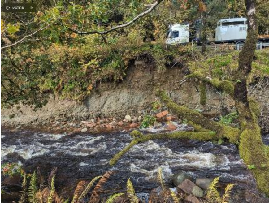
A83 Furnace Bank Erosion
