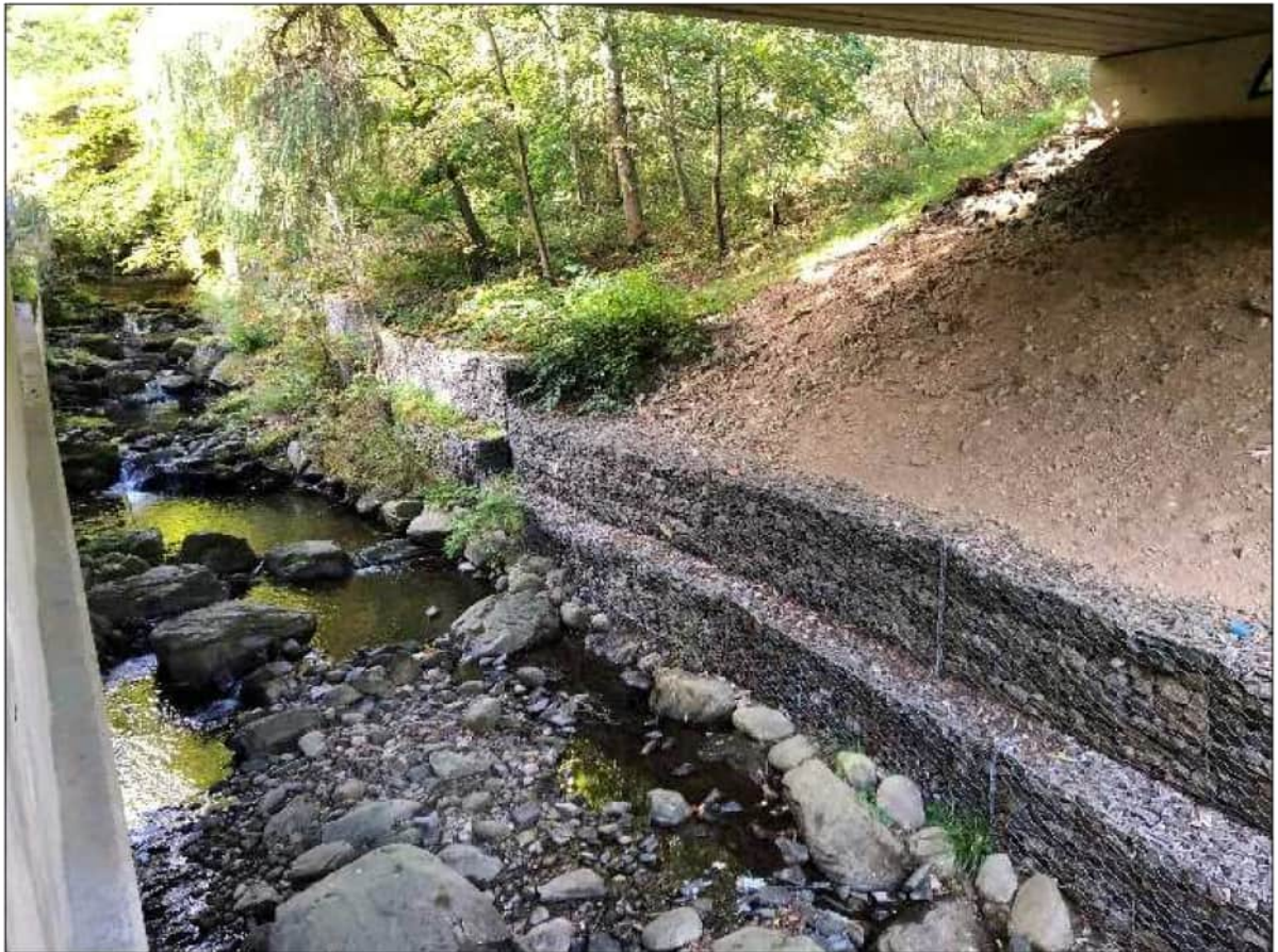
Photograph 3: Inchevan Burn – restored section beneath the existing A9.
