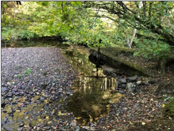
Photograph 1: Inchevan Burn – weir 900m upstream of existing A9 crossing.
