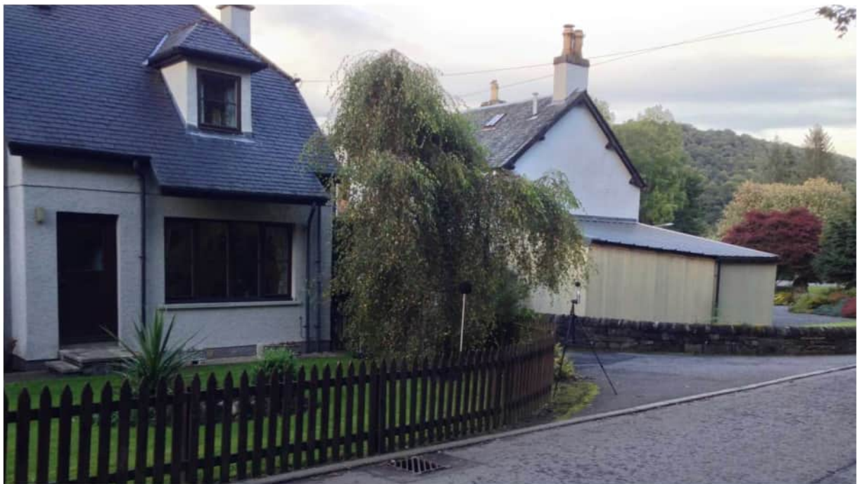
Photograph 7: Noise Monitoring Equipment at Corbiere
