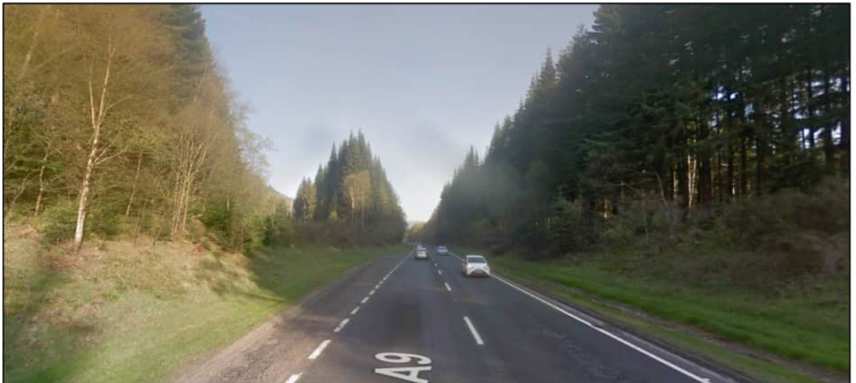
Photograph 6: Lay-by 1 (Image from Google Street View captured April 2019 © 2021 Google)
