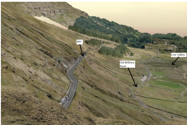
Plate A19.3.12 - Drone capture facing south, showing the A83, OMR and the hillside channels on the steep slopes of Beinn Luibhean above the Croe valley
