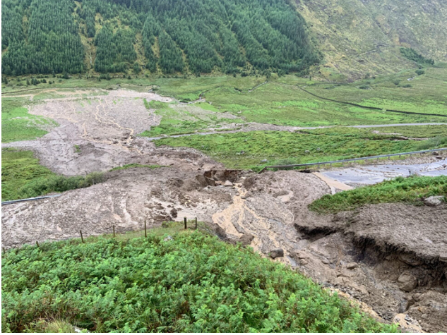
Plate A19.3.19 – Example of channel and overland flow crossing the A83 and OMR to the base of Glen Croe
