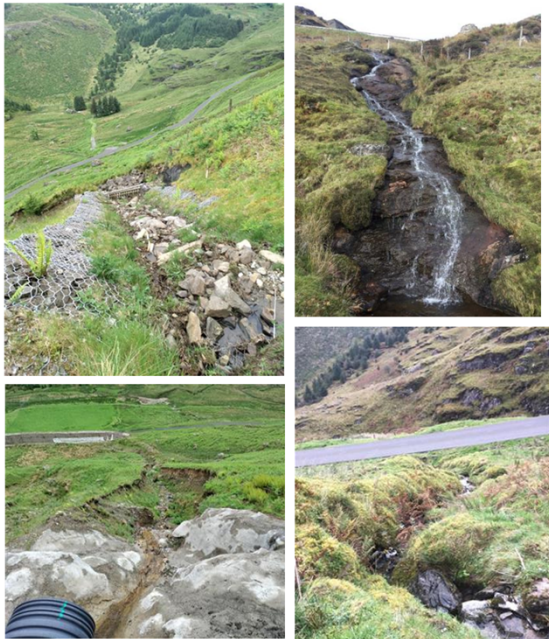
Plate A19.3.16 – Further examples of channels downstream of the A83
