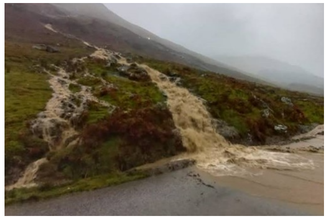
Plate 19.3.22 – Surface water flow spilling onto A83
