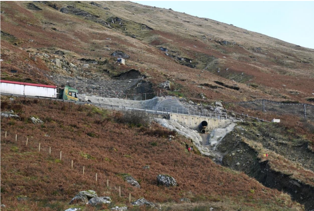
Plate 3 – Catch-pit and fencing works on the A83
