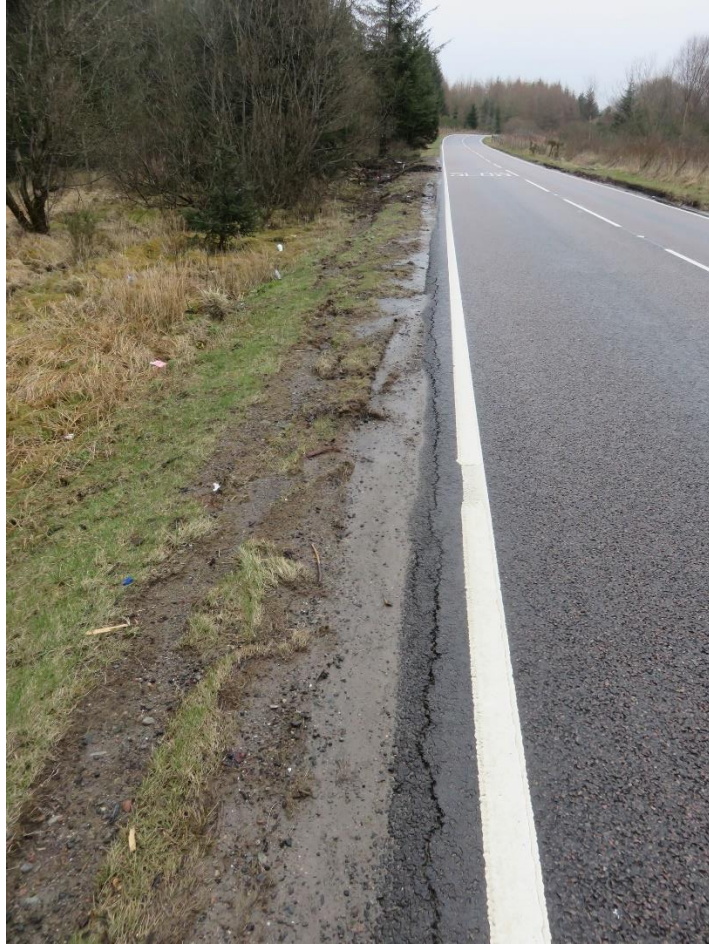
Figure 3-9 - HGV overrun on A82
