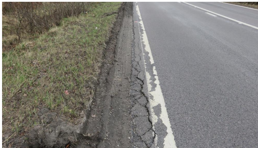
Figure 3-8 - HGV edge overrun on A95
