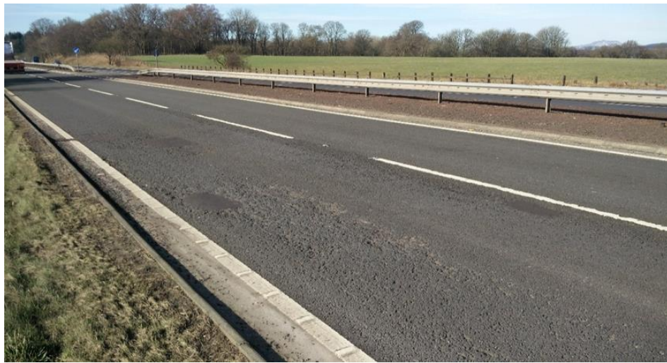
Figure 3-4 - VCS near A9 Dunblane in 2016, prior to treatment
