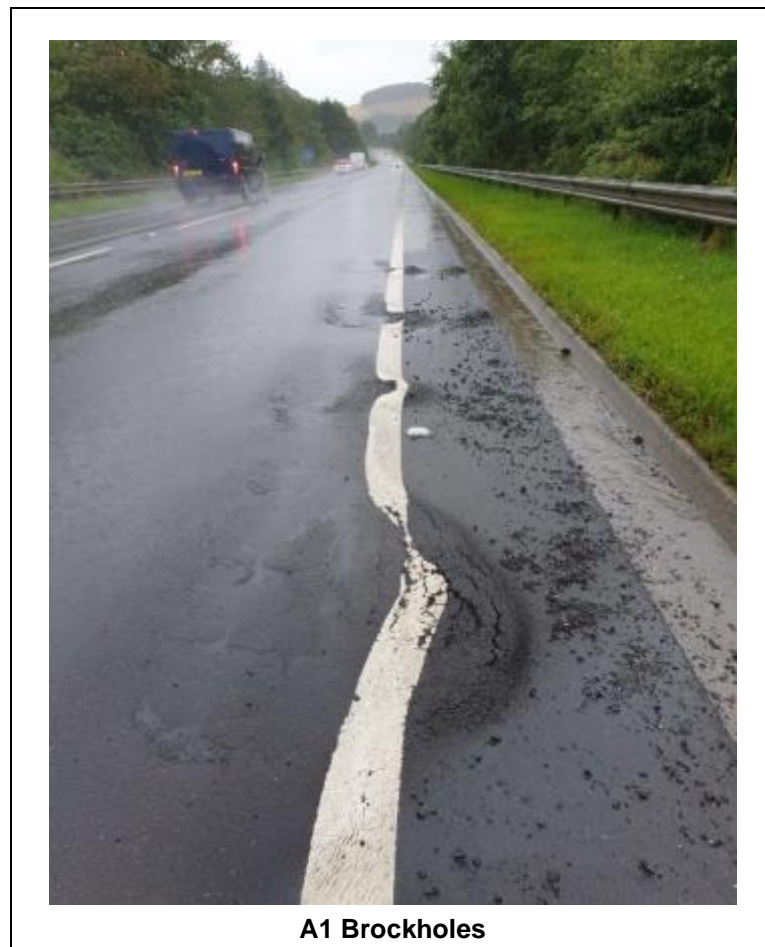
Figure A-2 - Early life defect in the SE
