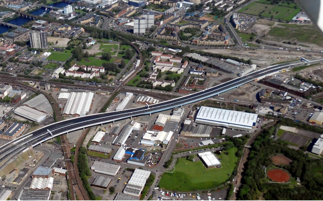
Figure 4.15.19.A – M74 2-1 80 Port Eglinton Viaduct
