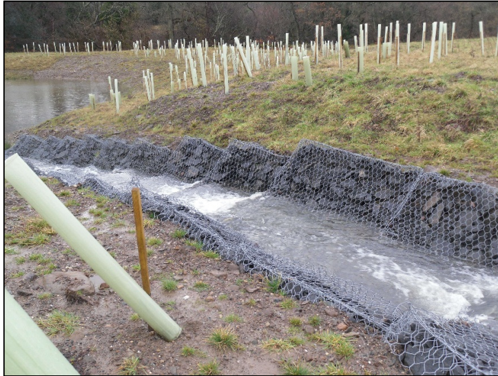
Figure 3 – Gabion channel between ponds
