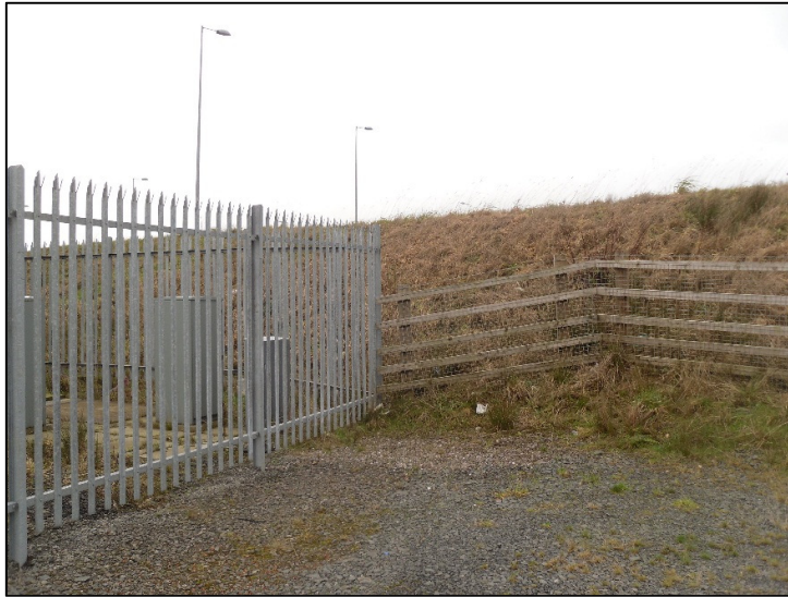
Figure 7 – Location of the end of the otter fencing and more open fence around the utility buildings near Dalshannon.
