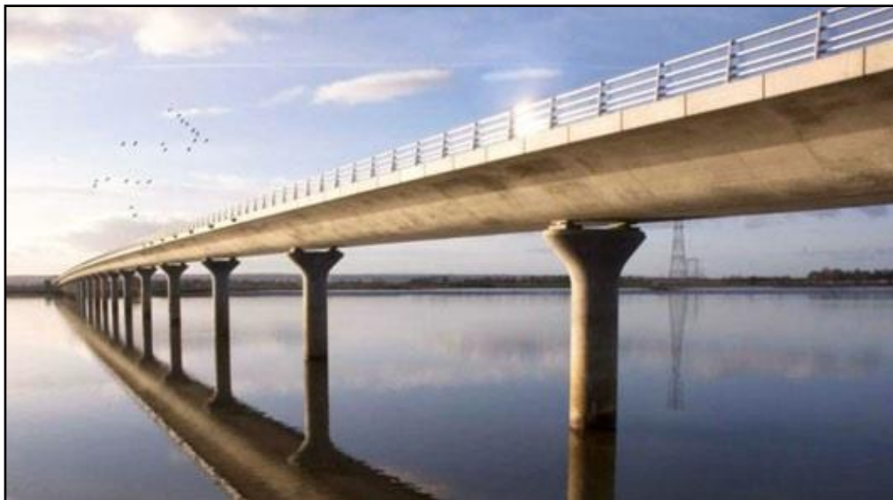
Figure 4.15.8.A - A876 50 Clackmannanshire Bridge
