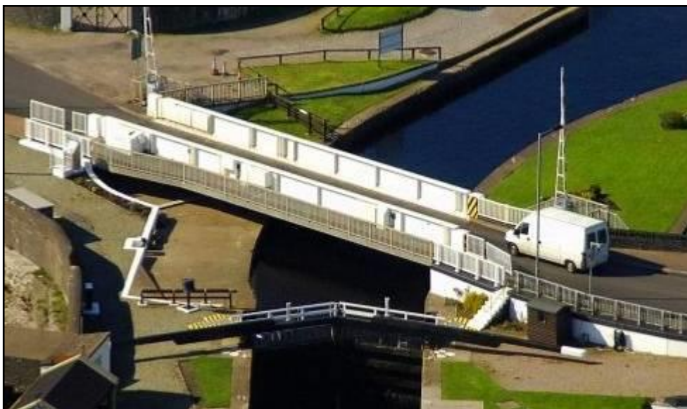
Figure 4.15.119.A – A83 240 Ardrishaig Swing Bridge
