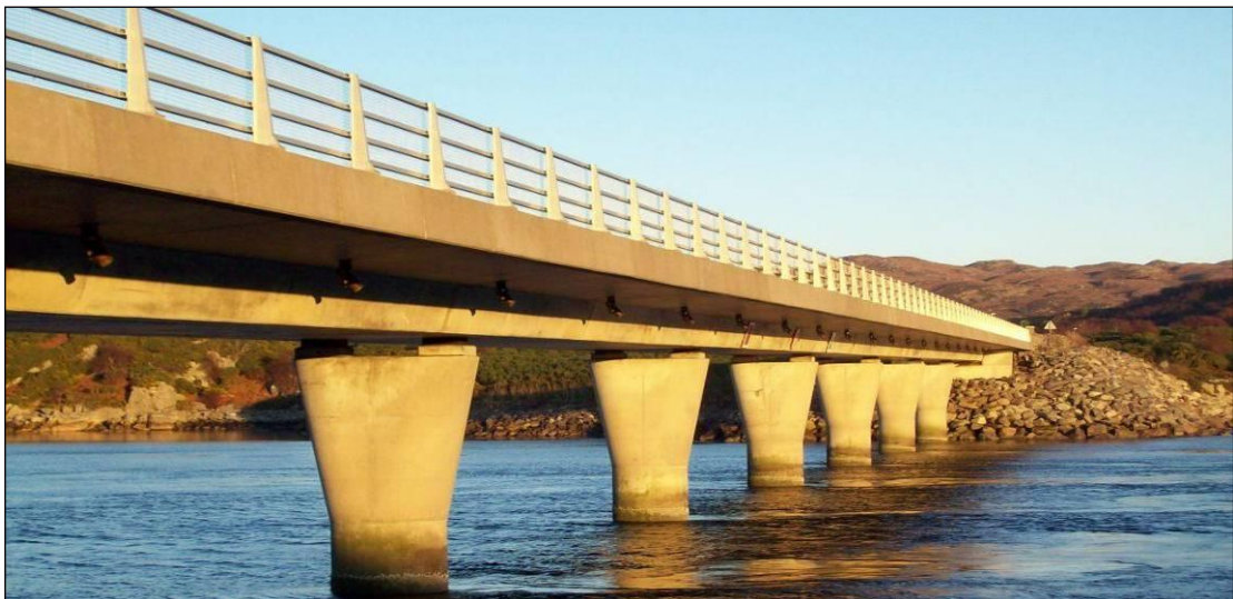
Figure 4.15.8.A – A87 280 Carrich Bridge
