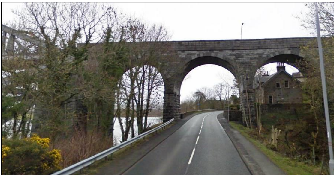
Figure 4.15.16.A – A828 9 Connel South Approach
