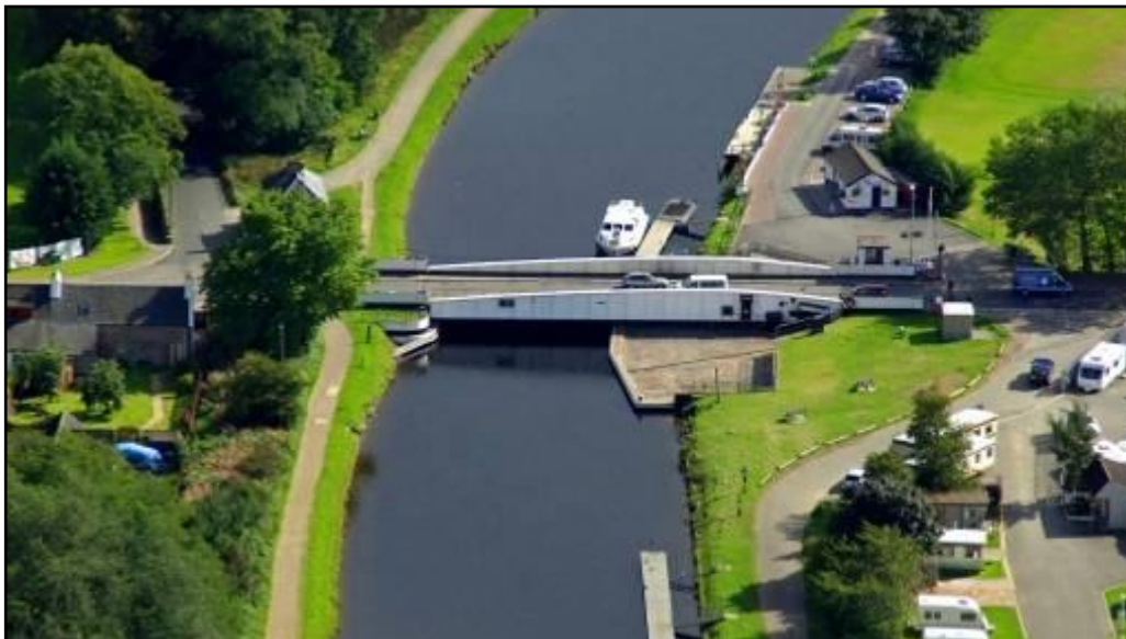
Figure 4.15.111.A – A82 1490 Tomnahurich Swing Bridge
