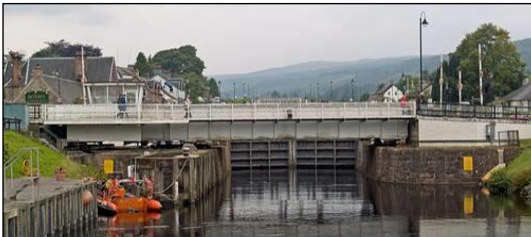
Figure 4.15.87.A – A82 1250 Fort Augustus Swing Bridge
